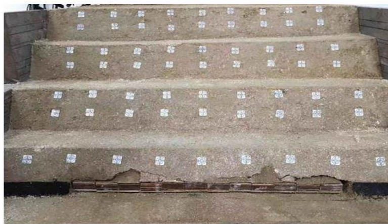
Figure 5. Displacement of slope mine wall in the second step of excavating coal pillars and paste backfill mining.
